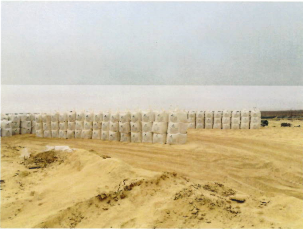
Stockpile of processed material awaiting sale and delivery
