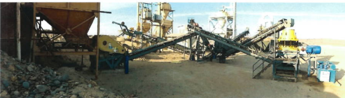
New installed plant with older equipment still utilised in background
